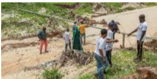
Effects of erosion in Sankandi Village, LRR
